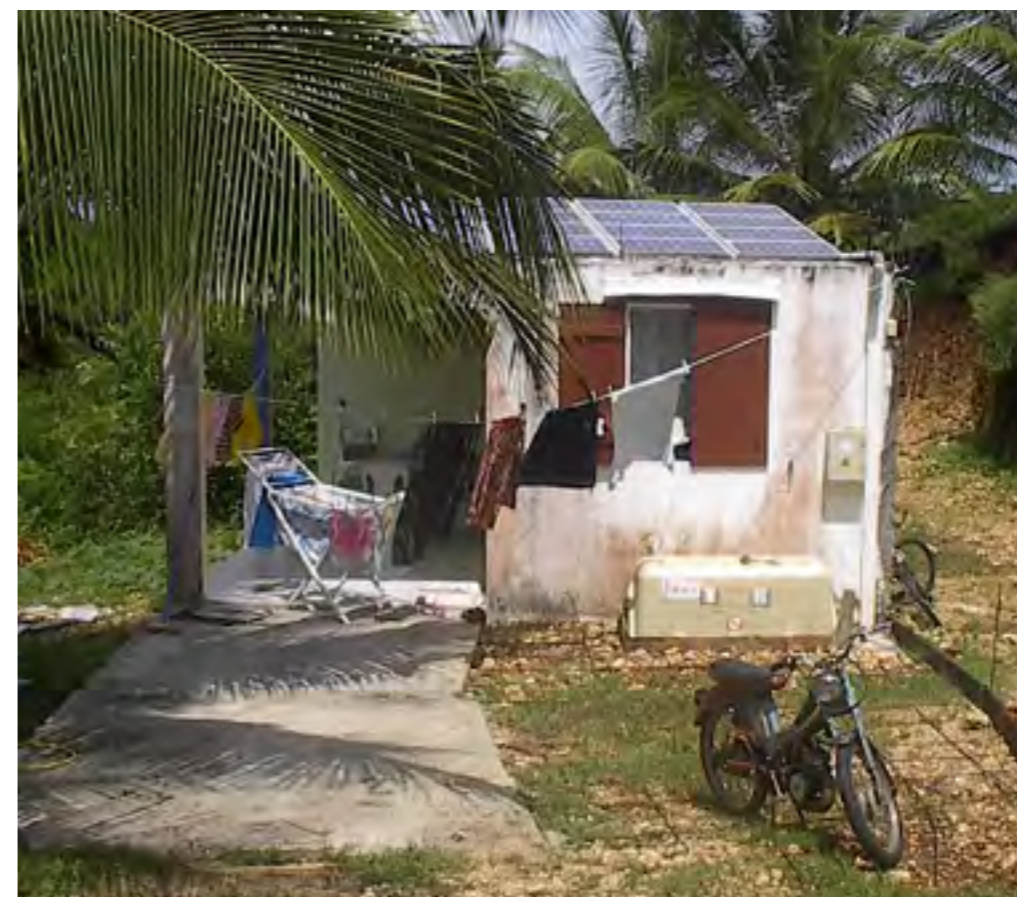
Construction illicite - Sainte-Anne
