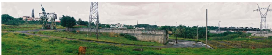
FIGURE 22: CENTRE DE TRANSFERT DE BLACHON, SOURCE CATRAM
