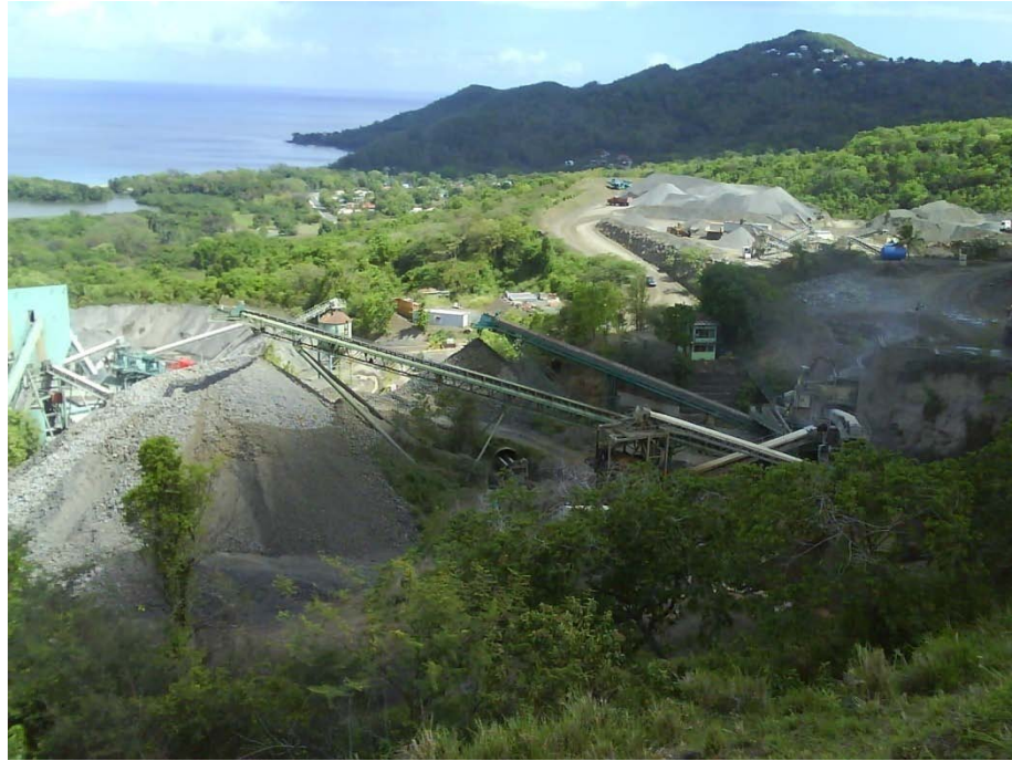
FIGURE 57: CARRIERE DE DESHAIES, SOURCE JONCTION
