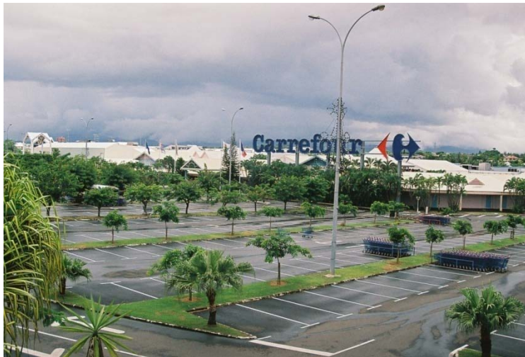
FIGURE 62: CARREFOUR DESTRELAND A BAIE MAHAULT, SOURCE CATRAM
